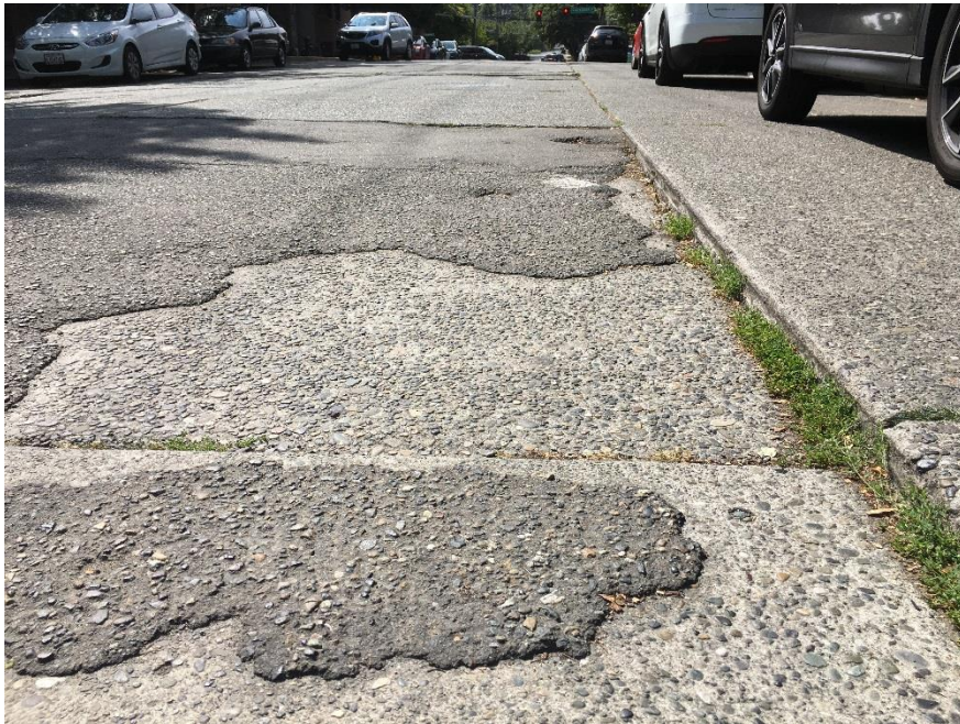
Figure 3: Close Up on the Panel Settlement in the North Section
