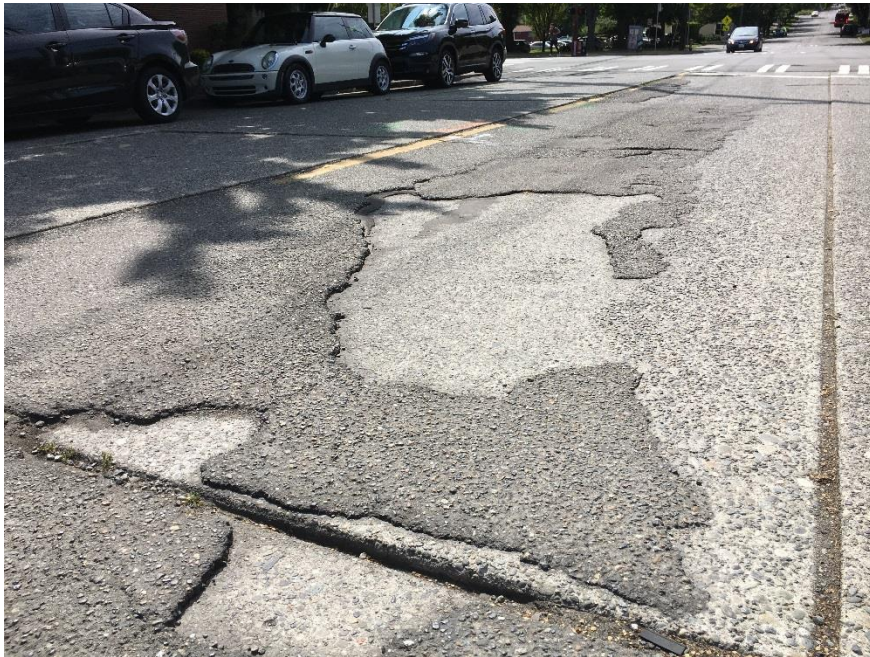
Figure 8: Close Up on the Panel Settlement for the South Section
