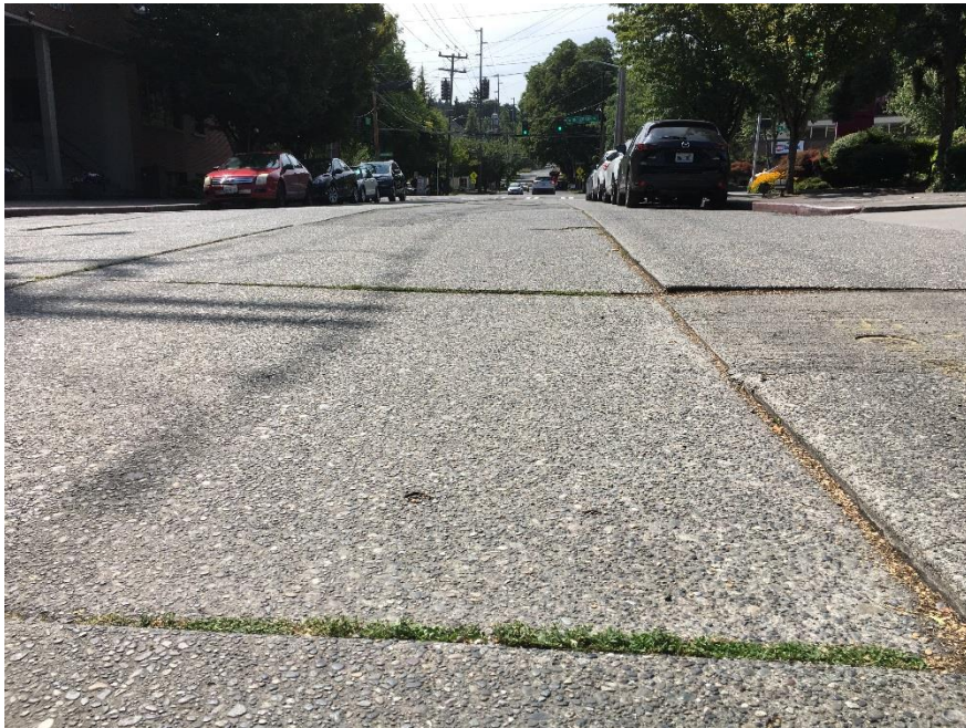
Figure 5: Close Up on the Panel Settlement for the Middle Area
