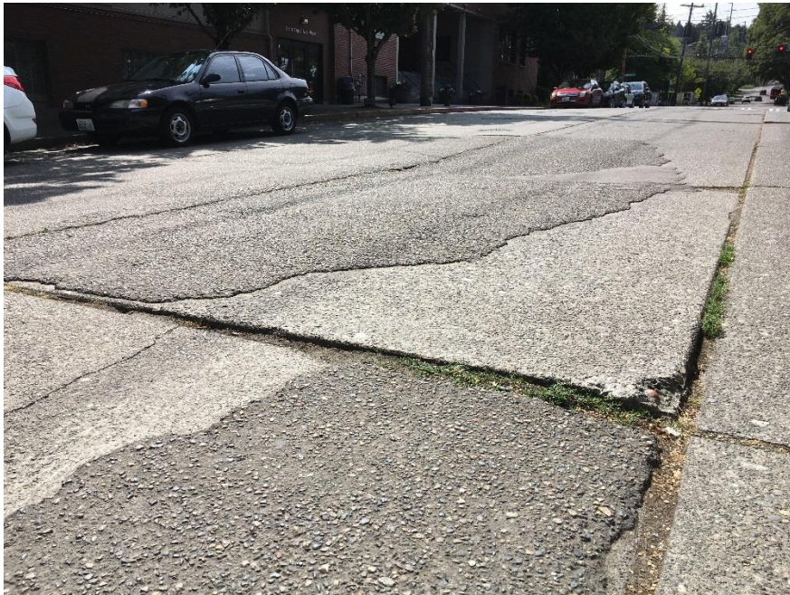
Figure 4: Middle Section Facing South
